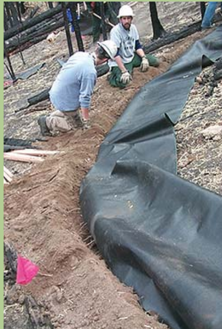
Example of silt fence installation
